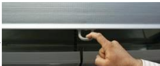
Using night curtains outside of working hours provides significant energy savings
